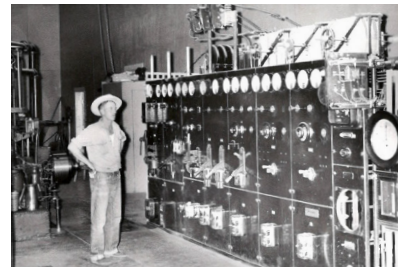
Willard Switch Board
